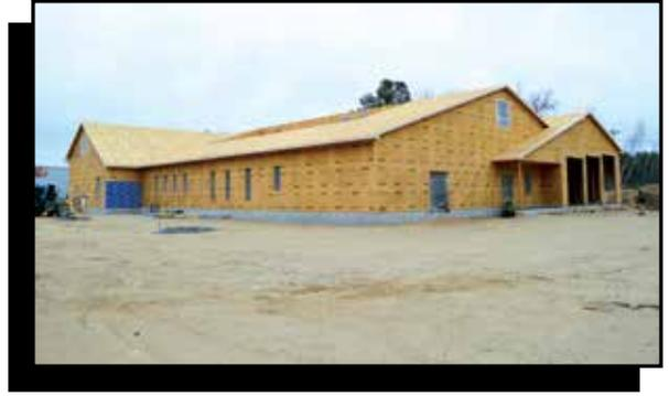
heating system in the attic. The trades were able to complete 90% of the work in the attic prior to the slab being poured, thanks in part to a 6-foot-wide catwalk that ran the length of the building. Windows and siding have been installed and work began on the interior metal stud and drywall partitions.
