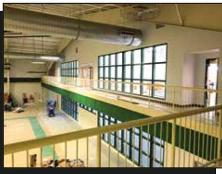
addition was all done using metal studs, as opposed to traditional wood framing. Although similar methods apply to both styles of framing, metal stud work pushed us out of our comfort zone for a little while, but we pulled through and completed the task on schedule.
